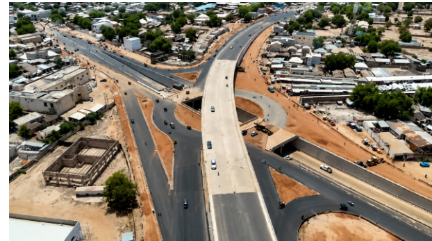
Construction of 3 level fly over and underpass at Damaturu
