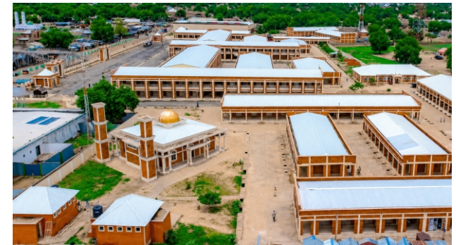
Construction of Damaturu Modern Market
