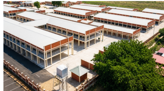
Construction of Gashu Modern Market
