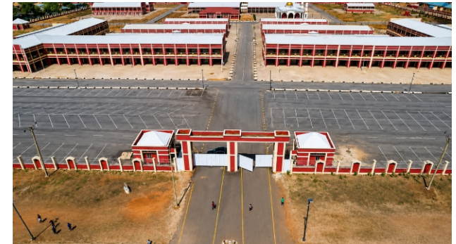
Construction of Nguru Modern Market
