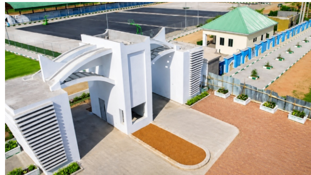
Renovation/ Construction of Damaturu Stadium
